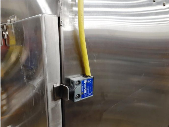
Door cut-off switch
