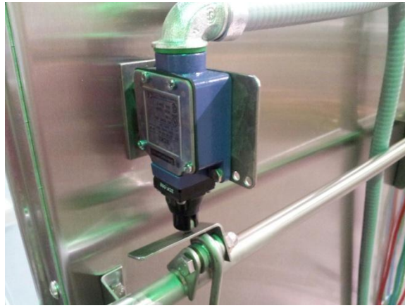
5-AGS Door cut-off switch and lever arm
