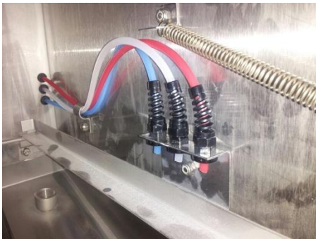
Showing chemical lines above sump
